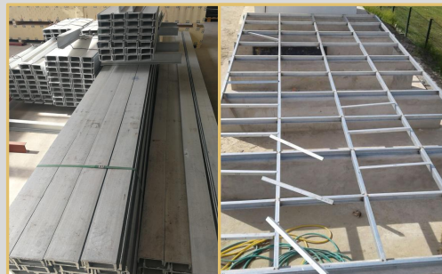
C-channel for base Q235B with HDG
